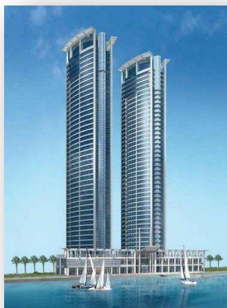
JULFAR TOWERS – RAK (B + G + 43 Typical Floors)
