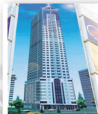
EMIRATES ISLAMIC BANK (G + 7P + HC + 37 Typical Floors)
